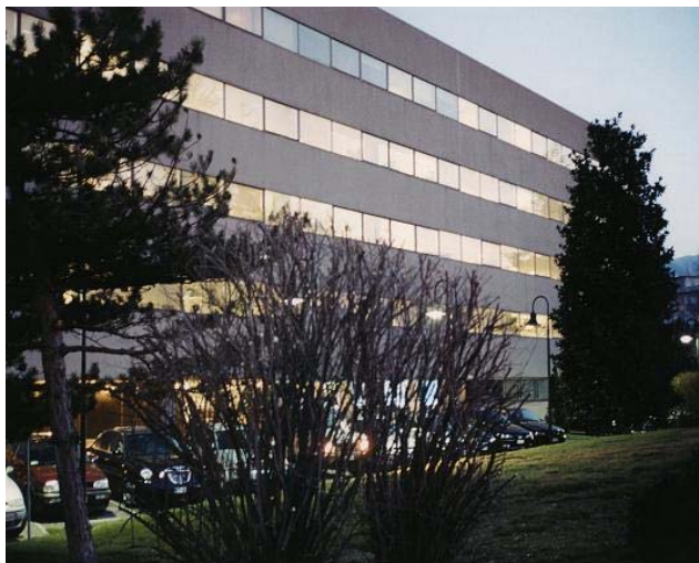
Ariston Thermo Group – Headquarters – Fabriano
